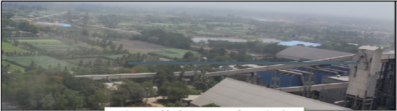
Covered belt conveyor from Coal storage area to Boiler
